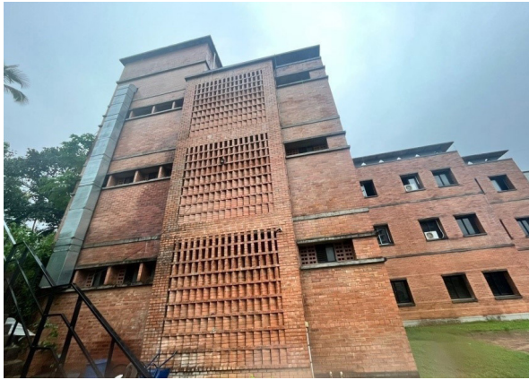
Figure 7 The Mashrabiya – locally made tiles with patterns that allow natural light and - panels embellishing the exteriors of the building
