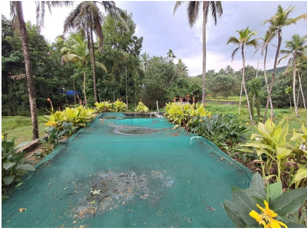
Figure 5 Constructed wetland enzyme based STP
