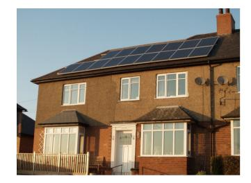
potential. The system also faced south over the Tyne Valley without any shading of any kind and was retrofitted to a roof of a building with a  $35^{\circ}$  pitch. The whole system cost £13,055 for installation. The results of the monitoring are shown in Table IV.
