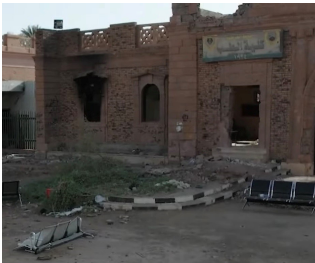
Figure 1: Structural damage of the Faculty of Medicine main entrance portico, Khartoum University
