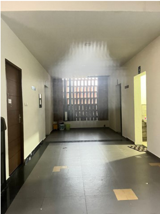
Figure 8 Layout styles save rainwater from splashing into the building while also ensuring natural cooling and airflow
