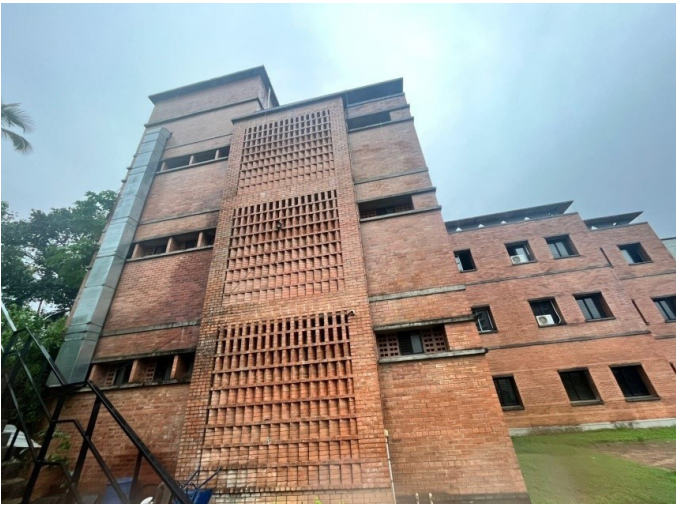
Figure 7 The Mashrabiya – locally made tiles with patterns that allow natural light and panels embellishing the exteriors of the building
